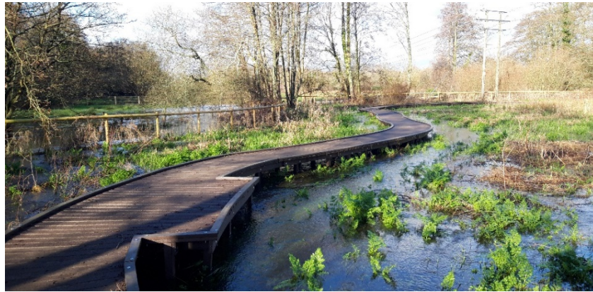
Examples of typical watercourse and floodplain crossings
